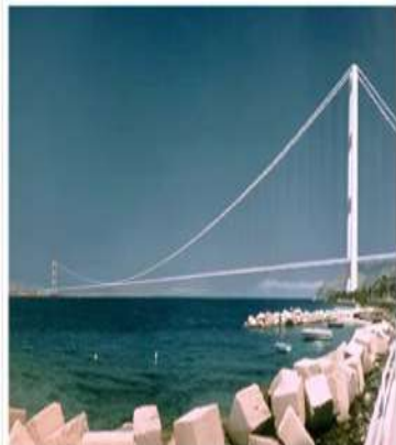
A 2001 simulation of what a bridge linking Italy's mainland with Sicily could look like. Photograph: AP
